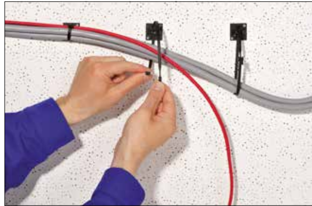
Q-ties can be used for both temporary and final cable installation.
