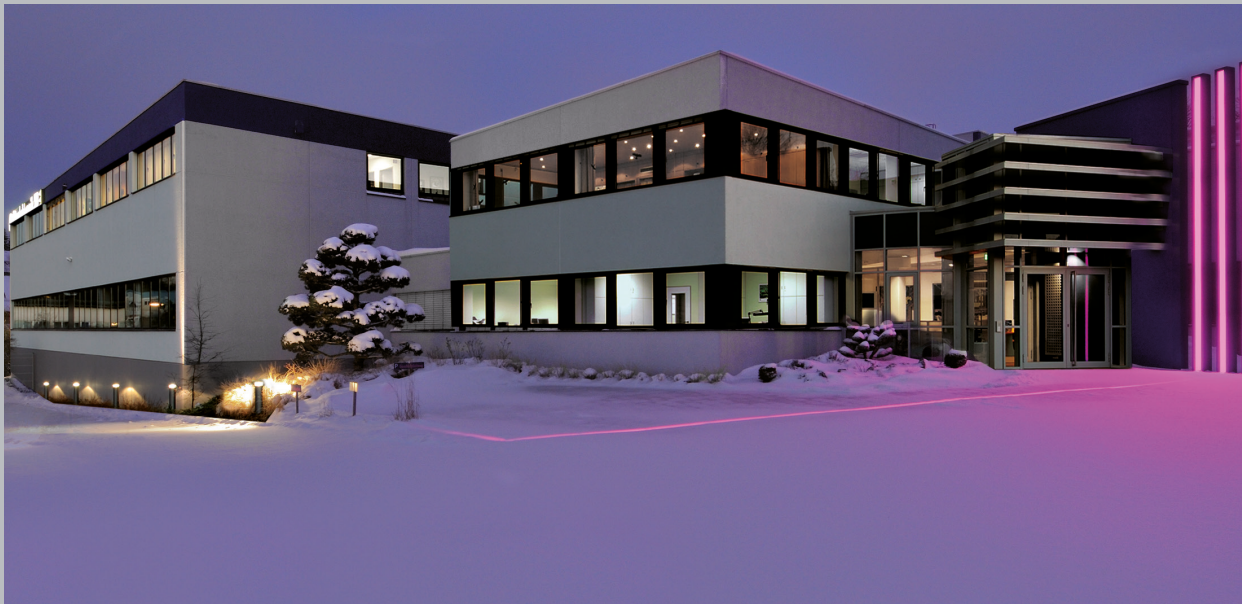
foyer of the company
