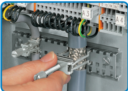
Addition of a shield (screen) clamping saddle.
