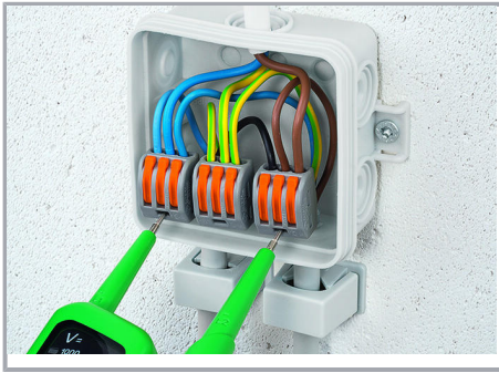
Testing via Profi-LED+ voltage tester (206-806).
