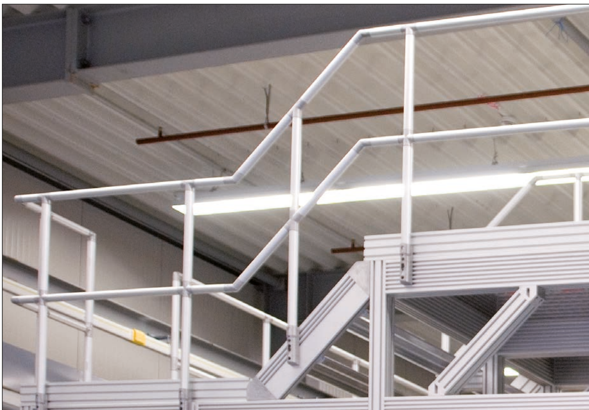
Staircase between two operating platforms.
