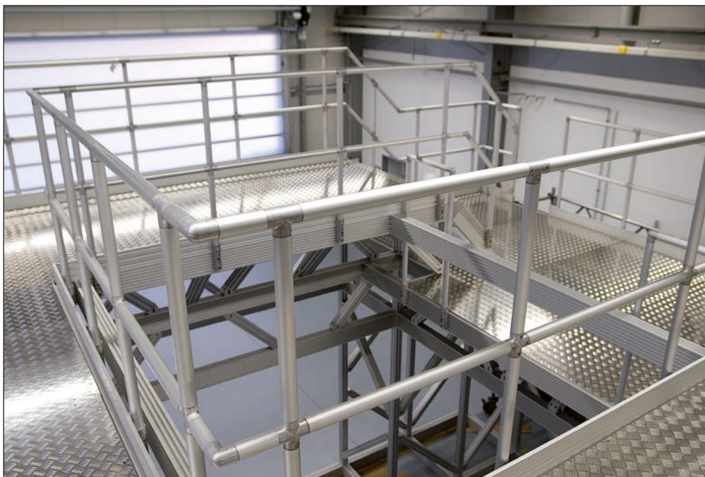
Working platform with ITAS railing
