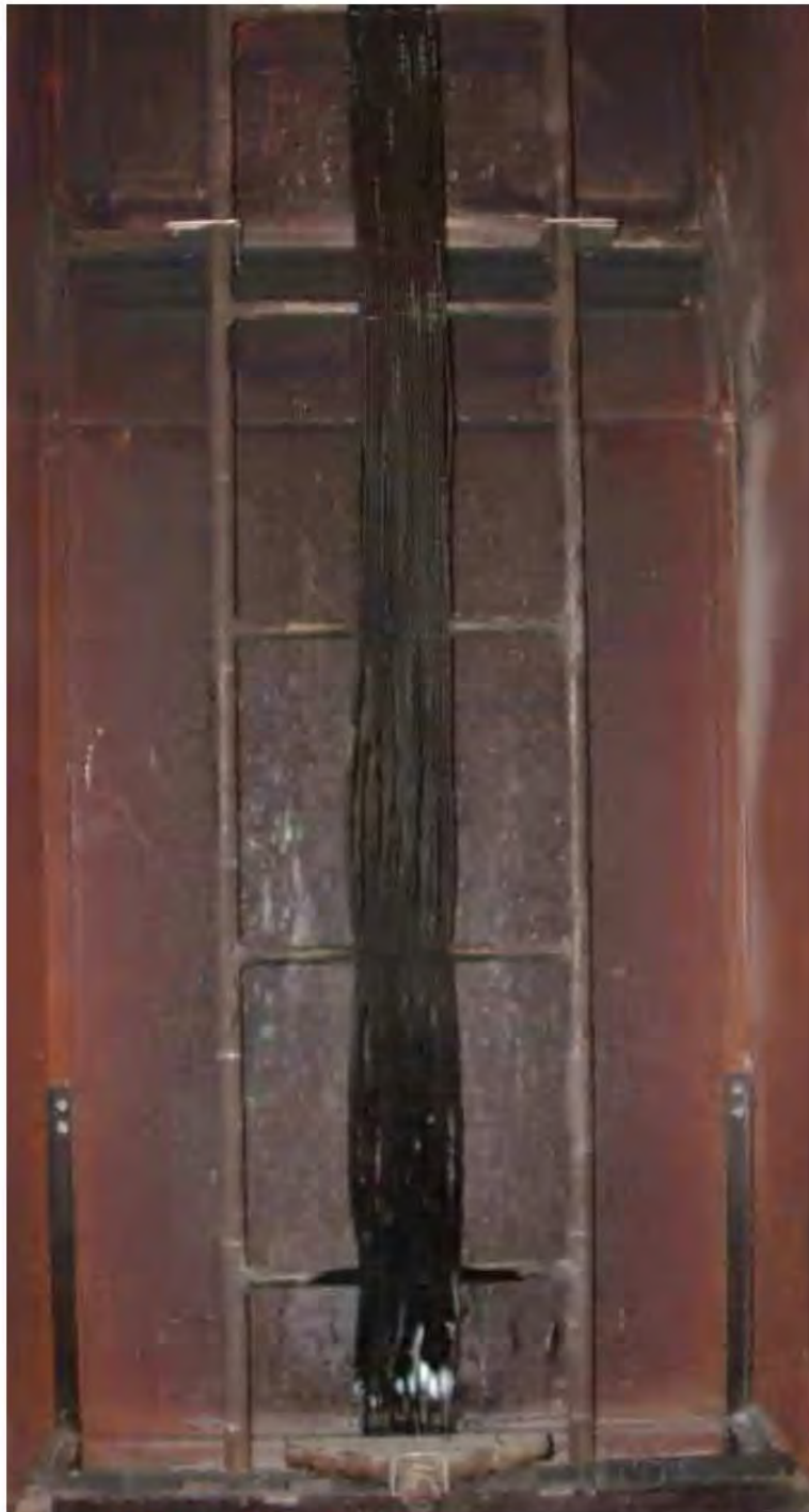
Photo 2: Cables after test.
