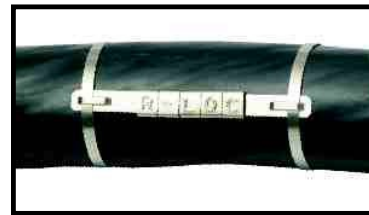
Marker Tags Installed on Power Cable
