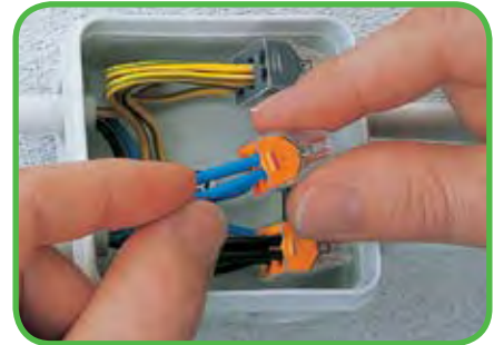
Wire removal Solid - Pull & Twist; Remove wire Stranded - Cut Wire; Discard connector Restrip; Insert wire in new connector
