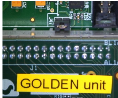
Figure 153: Jumper J47 Added Next to Golden Unit Socket
