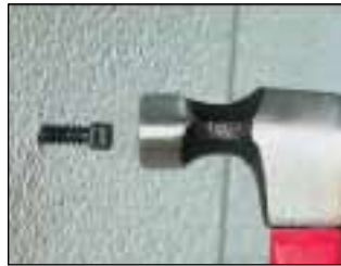
2. Hammer mount into hole.
