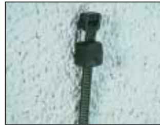
3. Place cable tie through mount.
