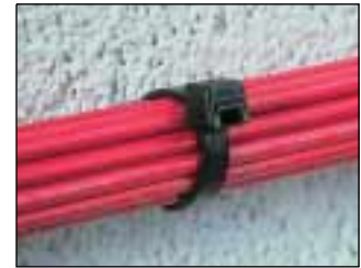
4. Install wires or cable.
