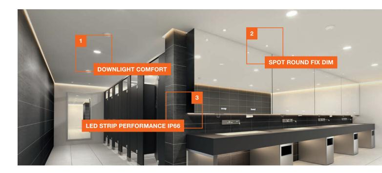
The mixture of indirect diffuse and directional light creates a pleasant atmosphere in washrooms and toilets. Uniformly bright general lighting throughout all sanitary facilities conveys a feeling of hygiene and cleanliness. For restrooms that are not permanently used, motion detectors are recommended which only switch on the light when needed.
