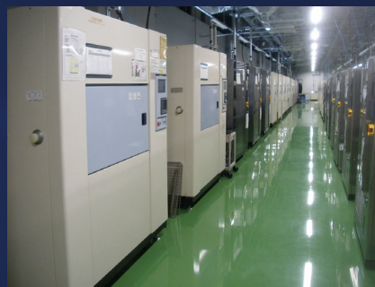
Evaluation equipment installed in the Integrated Evaluation & Test Laboratory
