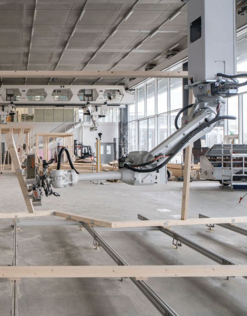
Copyright Roman Keller / NCCR Digital Fabrication.
