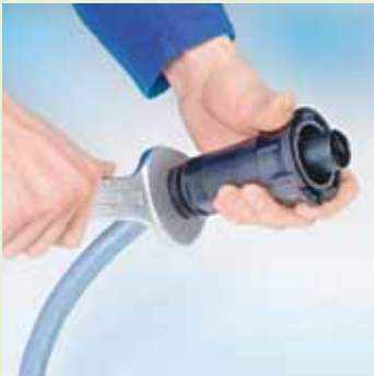
Tighten the gland using the required torque
