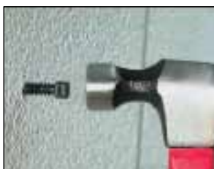
2. Hammer mount into hole.
